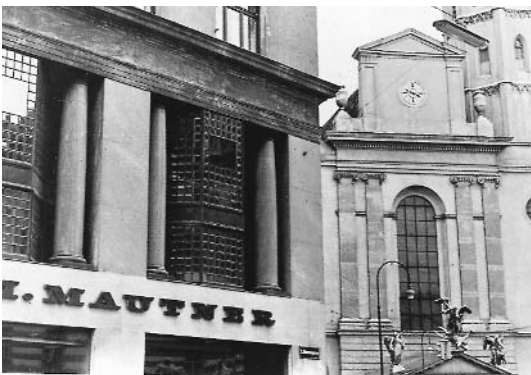
Adolf Loos, house on the Michaelerplatz, view of a detail of the Loos house together with the Michaelerkerche.
