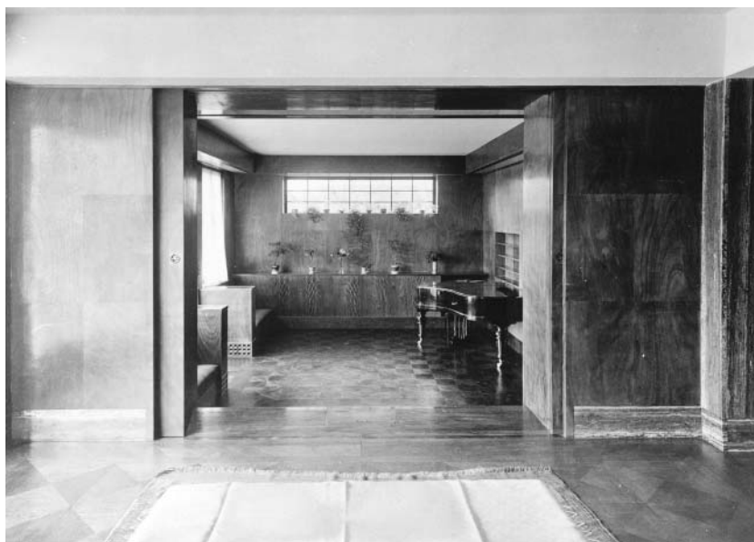
Adolf Loos, Moller House, music room seen from the dining room. (Photo: Albertina, ALA 2457.)
